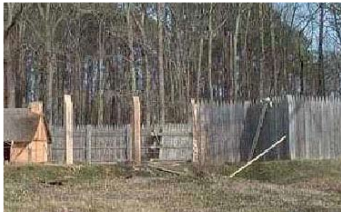
Building the re-created James fort, Jamestown Settlement
