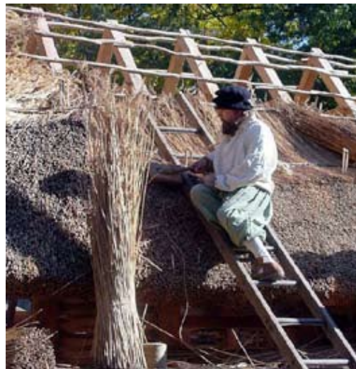
Thatching a roof in re-created James fort, Jamestown Settlement
